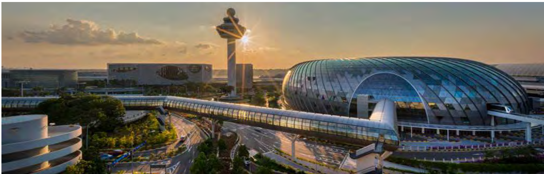
Source: Changi Airport Group
