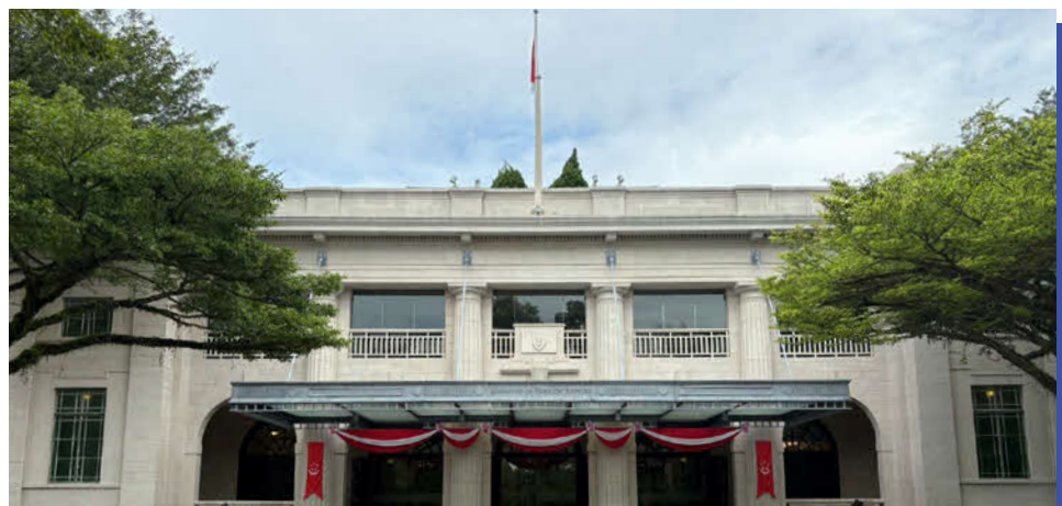
OTOM's restored facade after water-repellent treatment.
