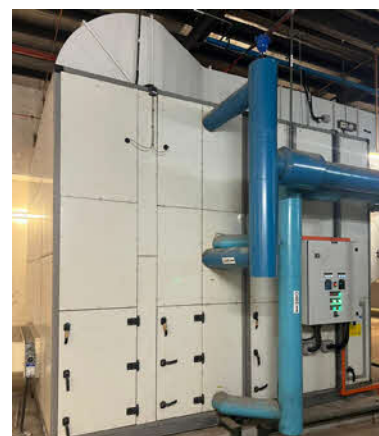
Replaced air handling unit ("AHU") at Blk 27.
