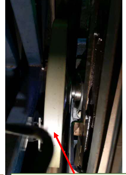
New Handrail Sheave.
