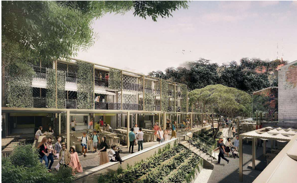
The former staff quarters will be fitted with lightweight timber and steel exoskeletal structures that not only function as vertical green walls to improve thermal comfort but also serve as external walkways that overlook a central food street © Homestead Holland Pte Ltd
