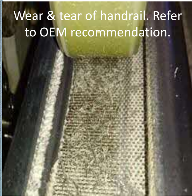
Clean up the foreign particles under handrail.
