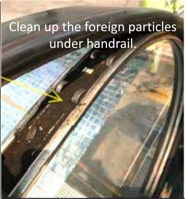
Wear & tear of handrail. Refer to OEM recommendation.
