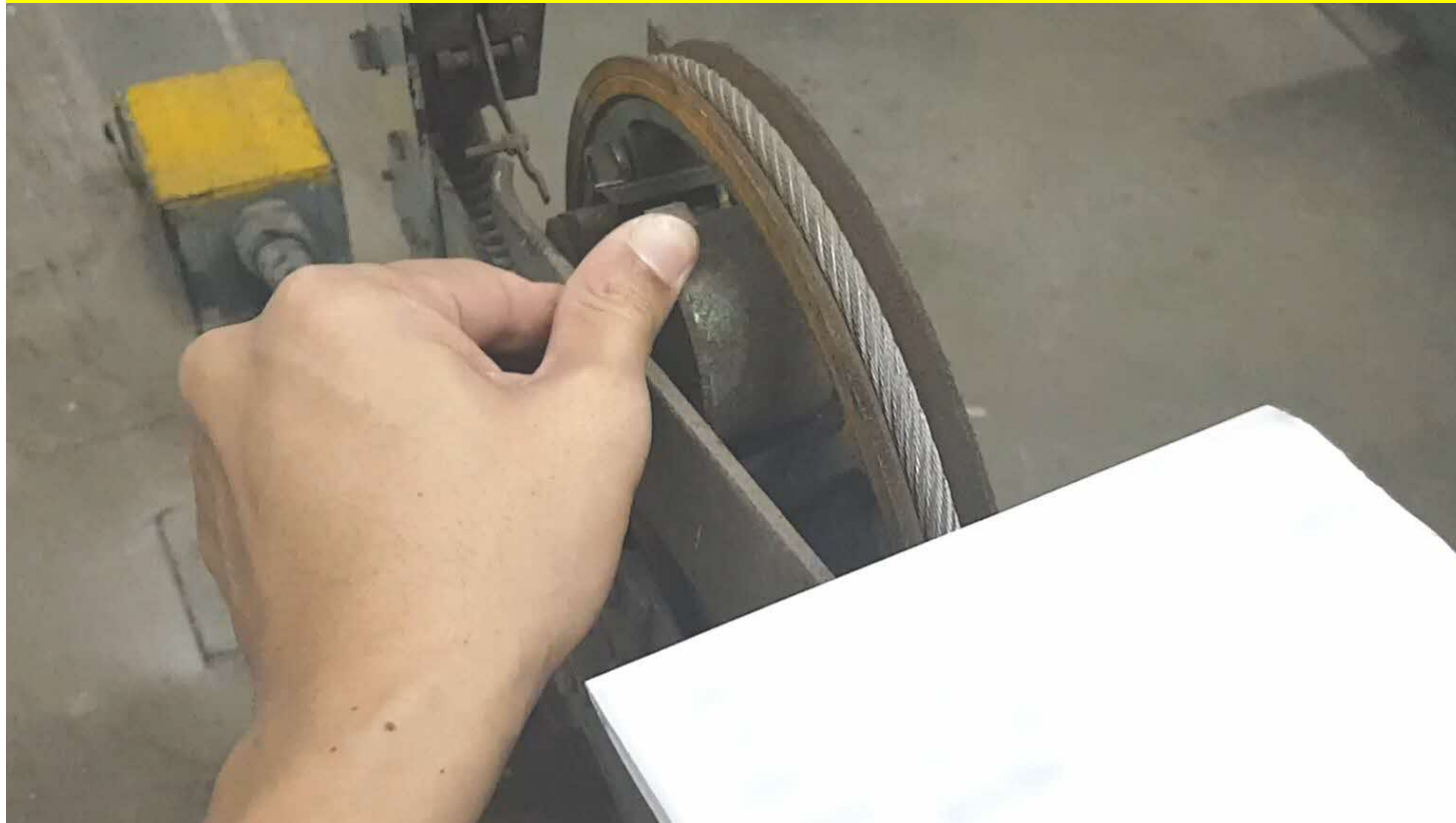
Video – Overspeed Gov. with restricted parts, not sufficiently lubricated.
