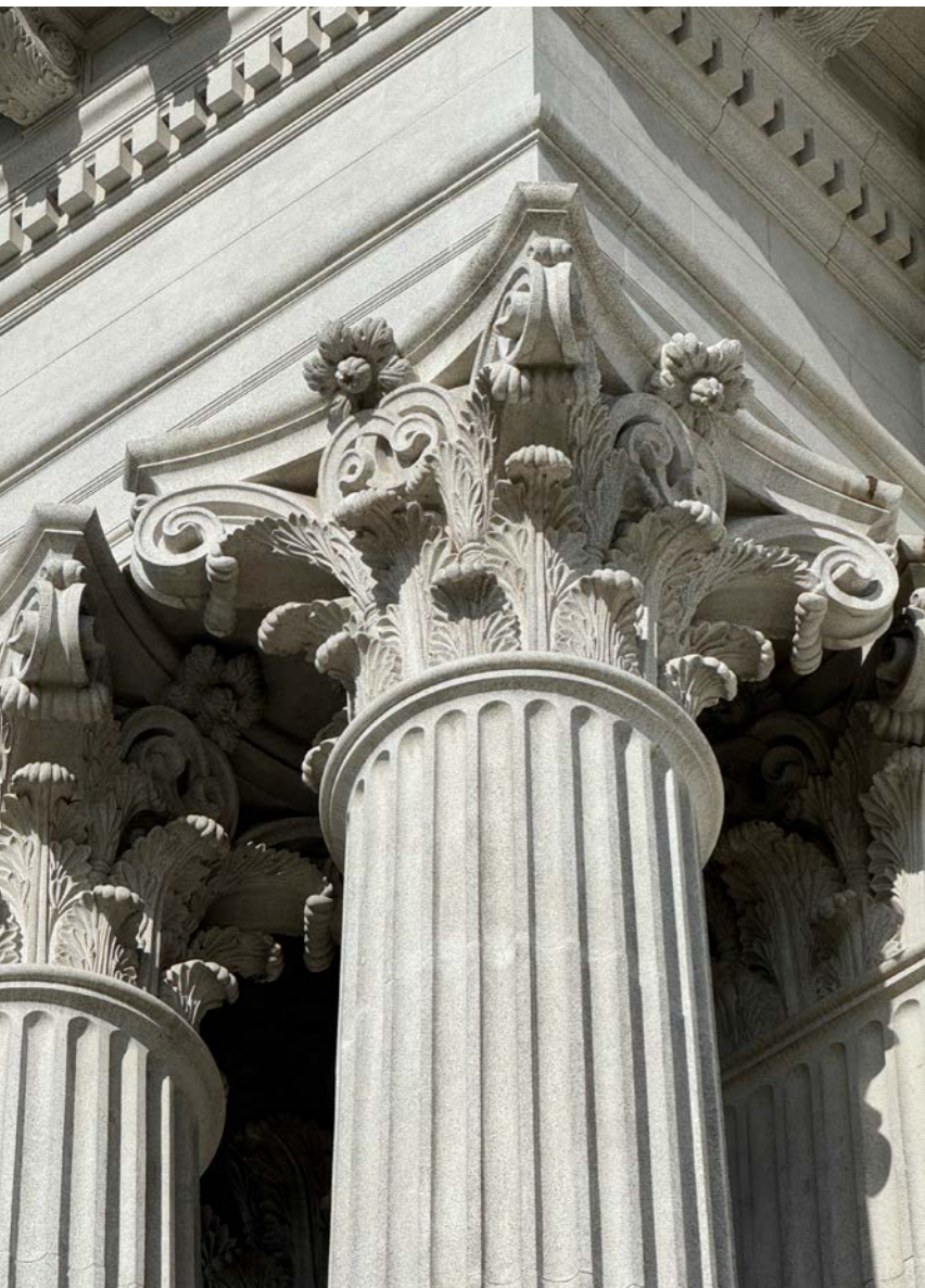
(Above) A closeup of the decorative work on the Corinthian columns of the former Supreme Court building, 2026. Photo by Jimmy Yap.
