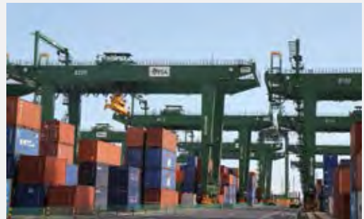
Automated & Remote Yard Cranes
