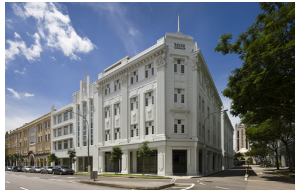
Top and bottom: Junction of Armenian Street and Loke Yew Street in 1992 and 36 and 38 Armenian Street in 2001.
