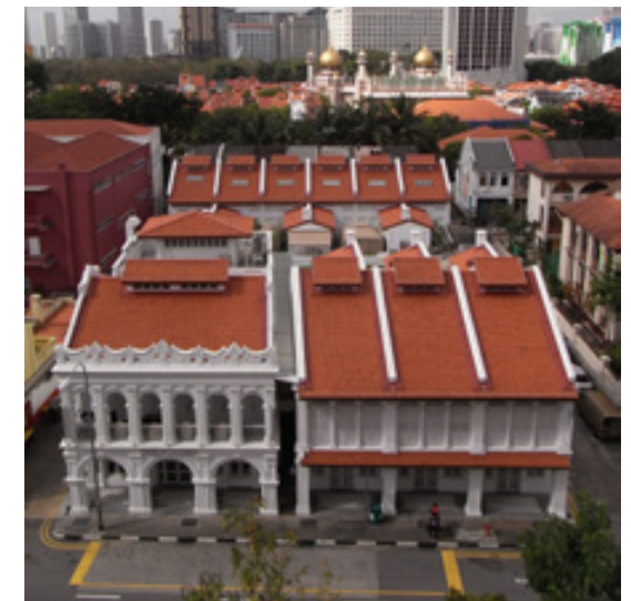
Two of the restoration projects by Towner Construction that won the Architectural Heritage Award - the Warehouse Hotel and 101 Jalan Sultan.
