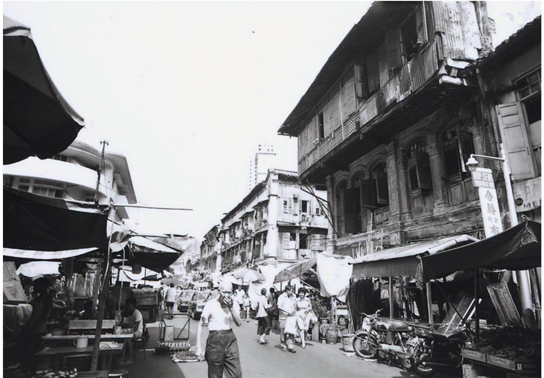
Smith Street in 1974. Erik Lorange noted in his 1962 report that the conditions of majority of residential buildings in the Central Area were "poor to a frightening degree."
