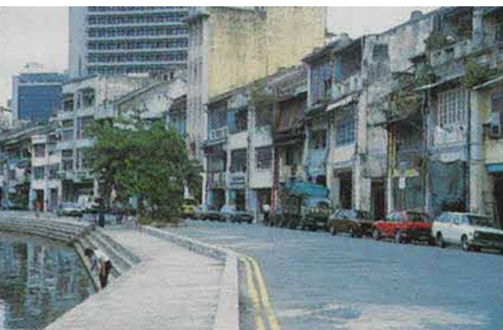
Original condition of the riverfront with service lane
