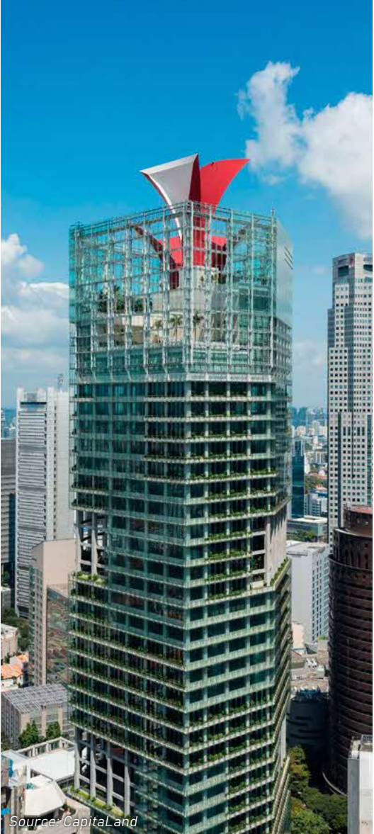
Source: CapitaLand Redevelopment of Market Street Carpark into CapitaGreen in 2014
