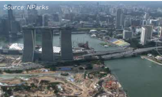
Construction of Gardens by the Bay
