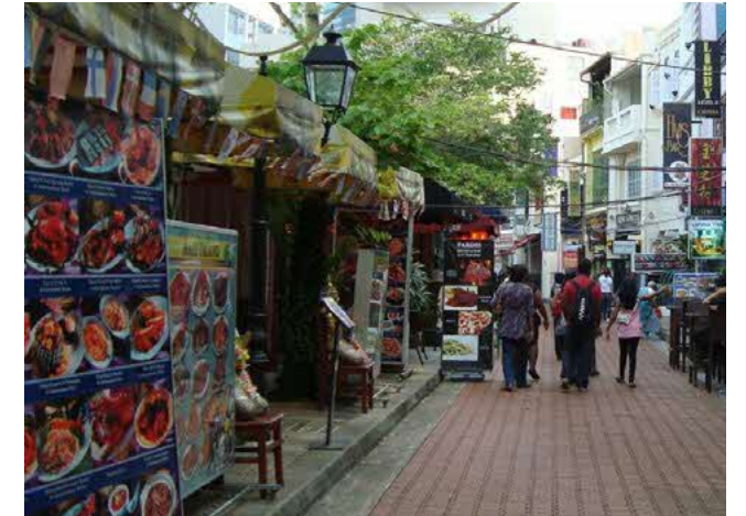
Unauthorised modifications over time which resulted in an unsightly promenade.
