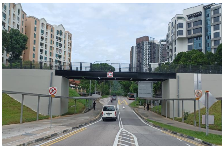
New Hillview Bridge (Credit: LTA)
