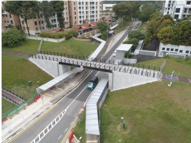
New Hillview Bridge (Credit: LTA)
