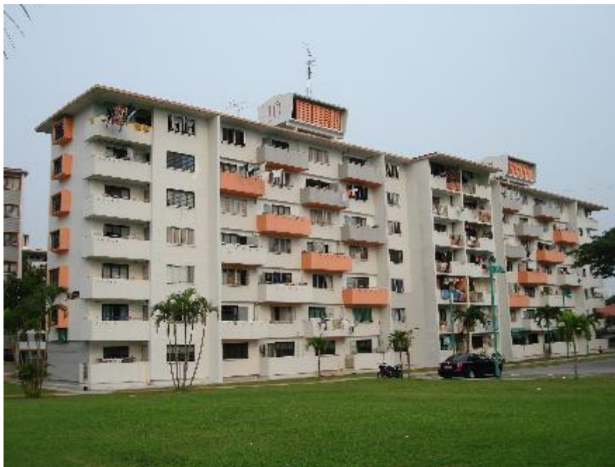
One of the seven-storey slab blocks designed with protruding balconies, a feature of tropical architecture Credit: URA
