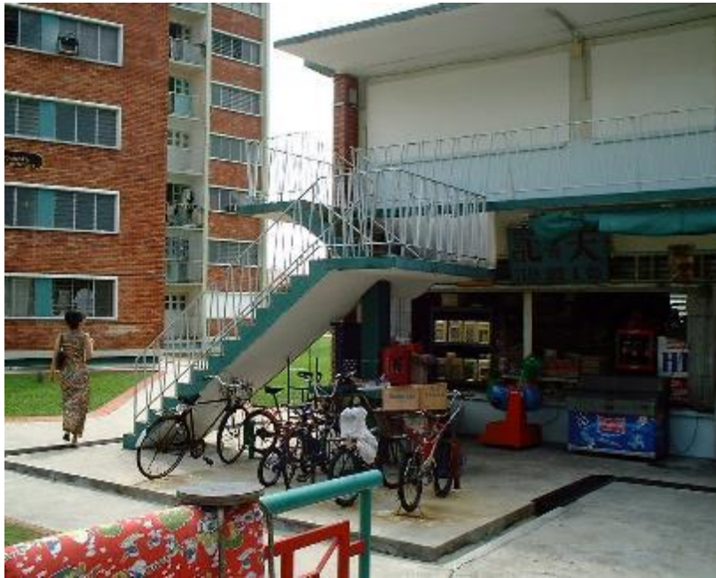
Block 12, a two-storey block, used to house shops serving the neighbourhood Credit: URA
