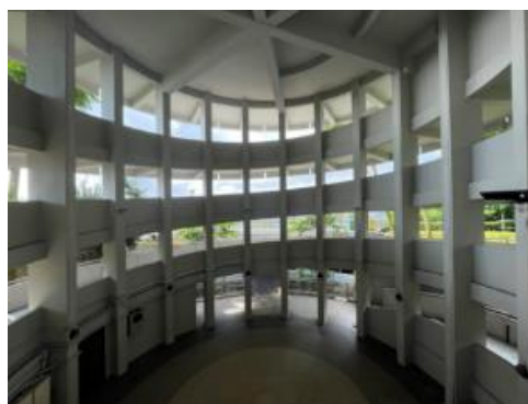
Unique spiral ramp supported by 18 columns
