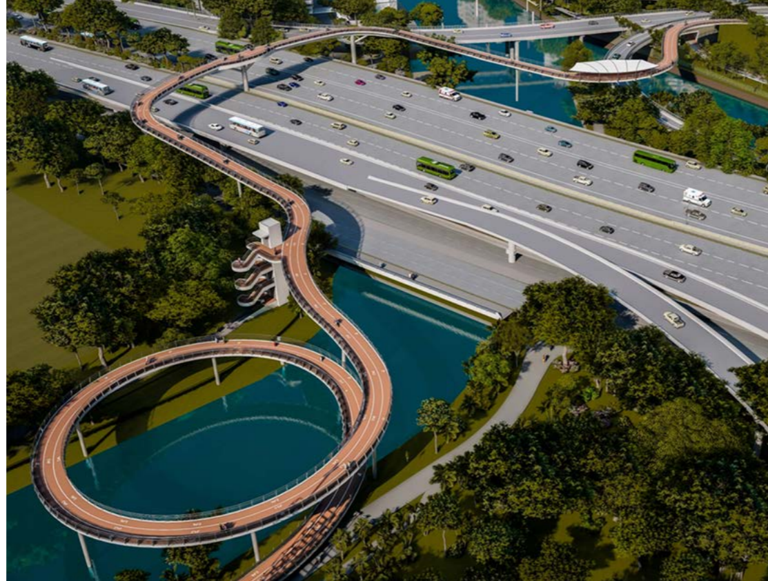
A 700m long elevated cycling bridge will be completed as part of the Bishan-to-city links, to bridge connectivity across the Pan-Island Expressway.
