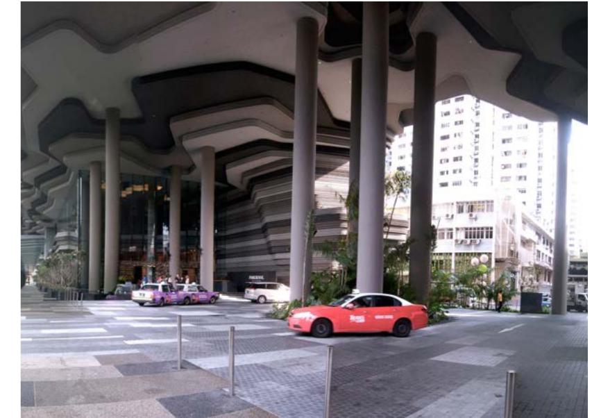
Main vehicular drop off at Park Royal Collection Pickering
