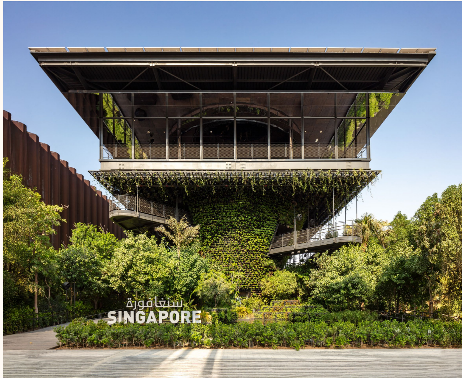
P*DA 2023 Design of the Year recipient — Singapore Pavilion Expo 2020 Dubai — is a successful prototype that shows how sustainable built environments could be designed for future cities. IMAGE CREDIT: URA
