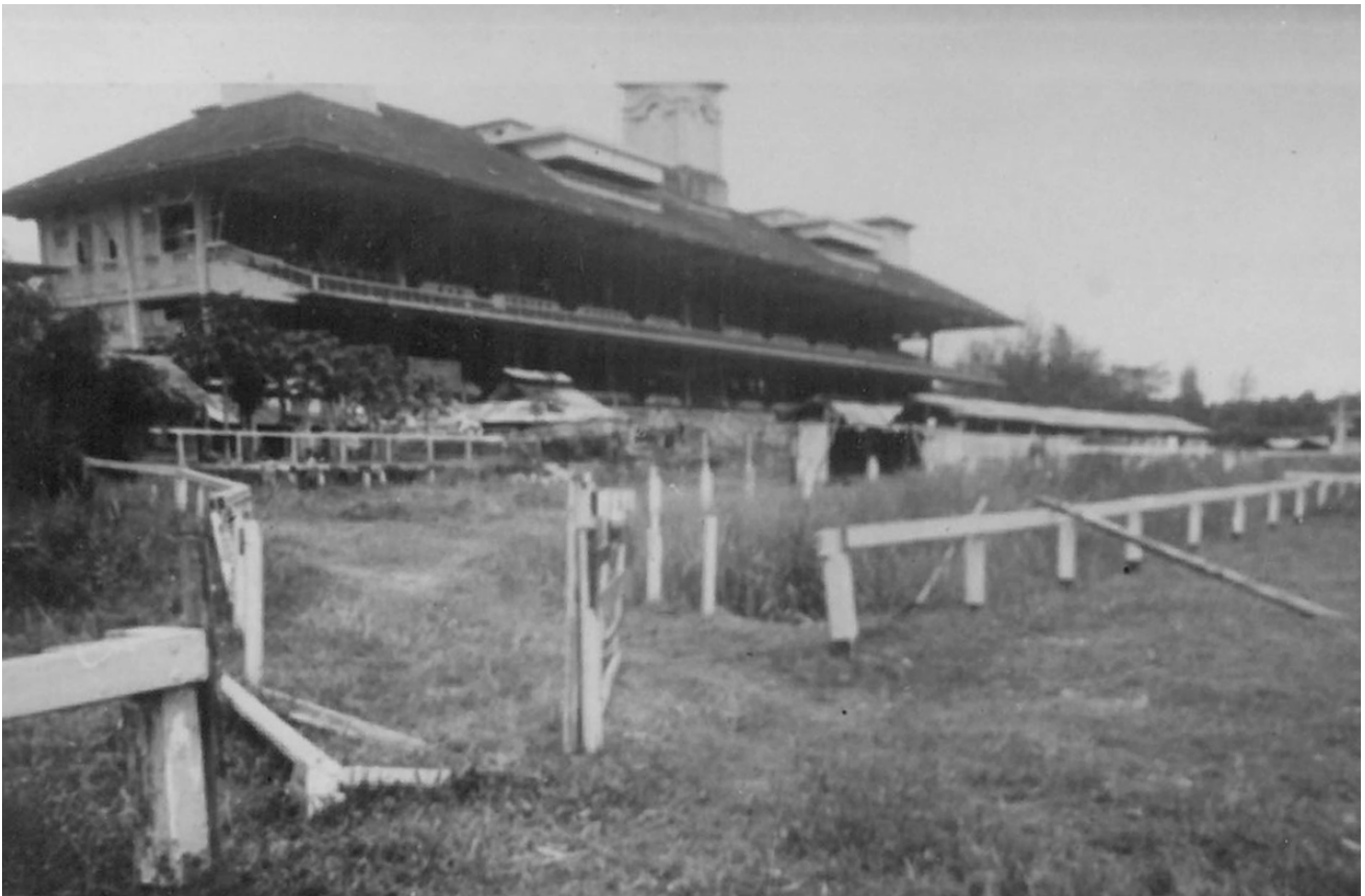
Figure 4.23 Post War view of South Grandstand. (Source: Mark Bailey)
