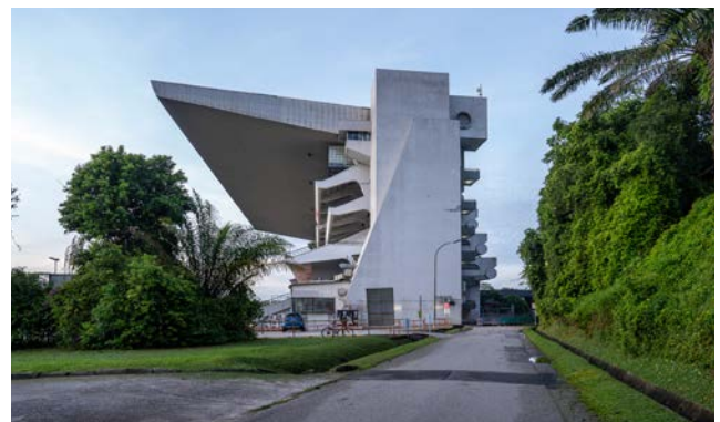
Figure 8.6: Existing view looking south to the North Grandstand.
