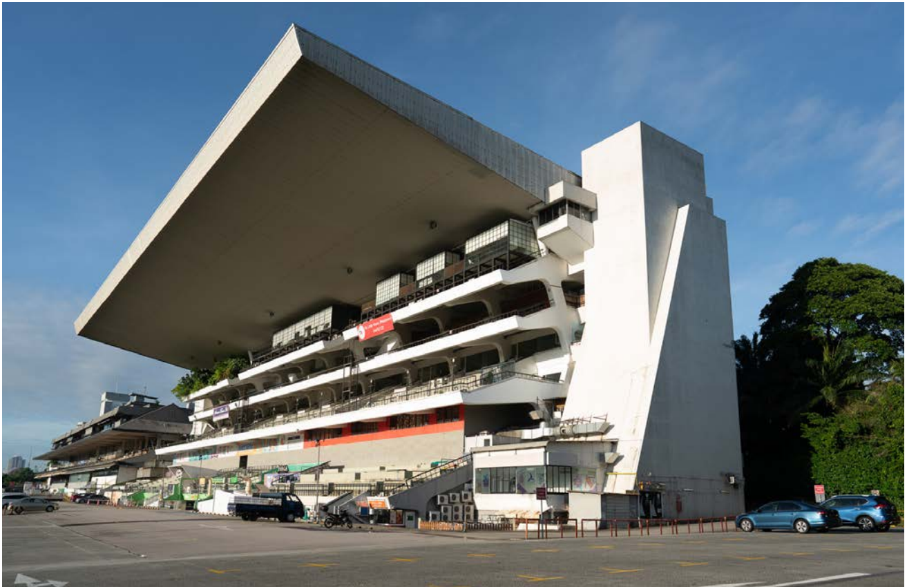
Figure 4.2 North Grandstand in 2021
