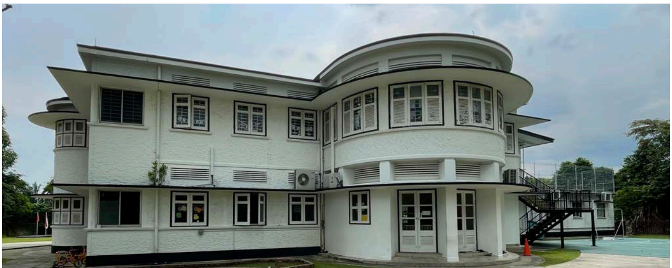
Top: Figure 4.10 Building No. 3 Bottom: Figure 4.11 Building No. 5
