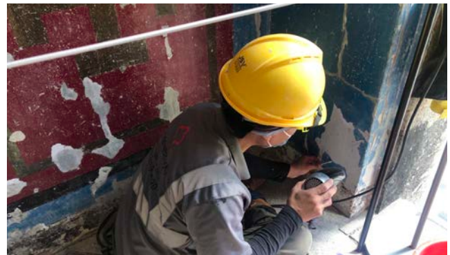
Figure 8.24: Conservation of paint layers in progress
