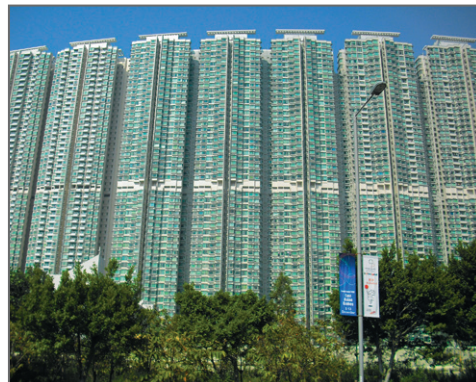
Figure 1: Wall-like developments in Hong Kong
