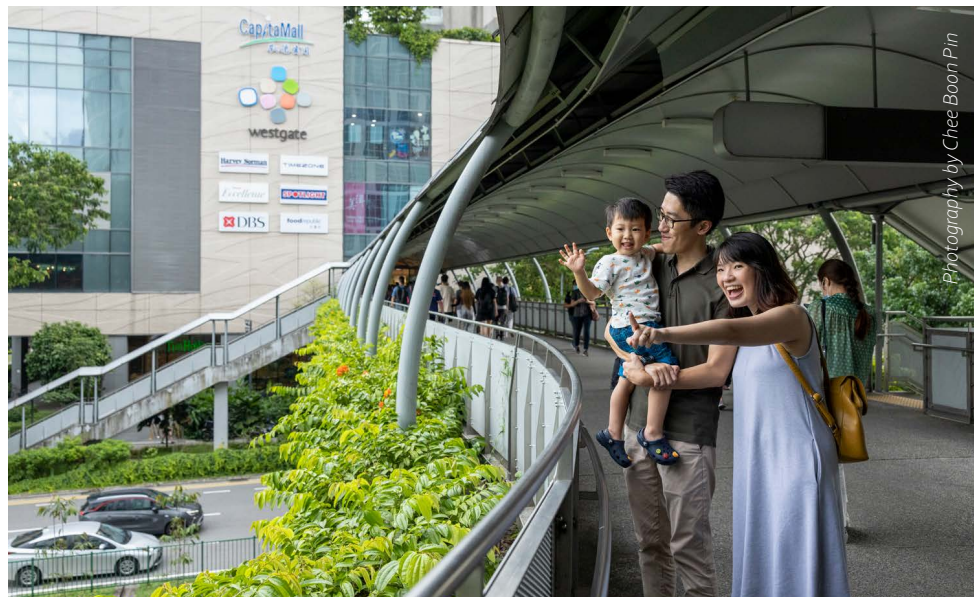
View of the J-Walk that connects Westgate and Ng Teng Fong General Hospital Jurong Lake District Planning and Urban Design Guide
