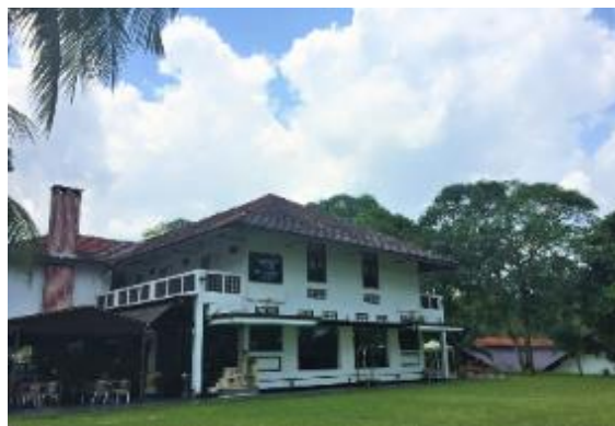
The two-storey building features chimneys on both the front and rear of the building, with wide roof eaves providing shade for the walkways along the side facades
