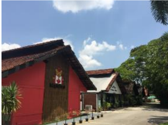
Four blocks of the horse stables can be retained and adapted for new uses
