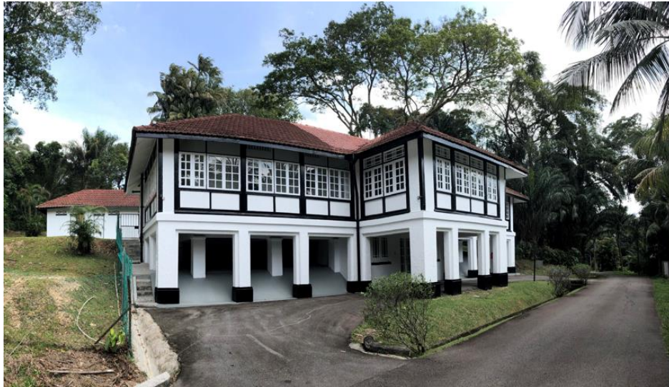
One-and-a-half storey bungalow of the Black and White typology, partially embedded in the slopes of the hill creating partial basements Credit: URA
