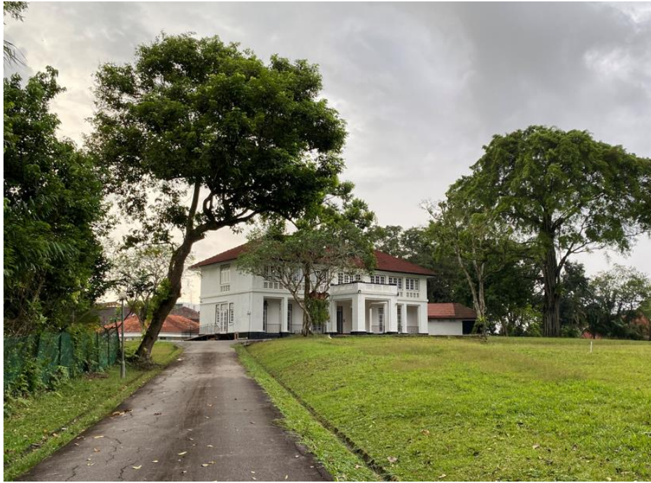
The estate is a largely intact pre-war British colonial bungalow clusters in Singapore, in terms of its topography, layout and building stock Credit: URA
