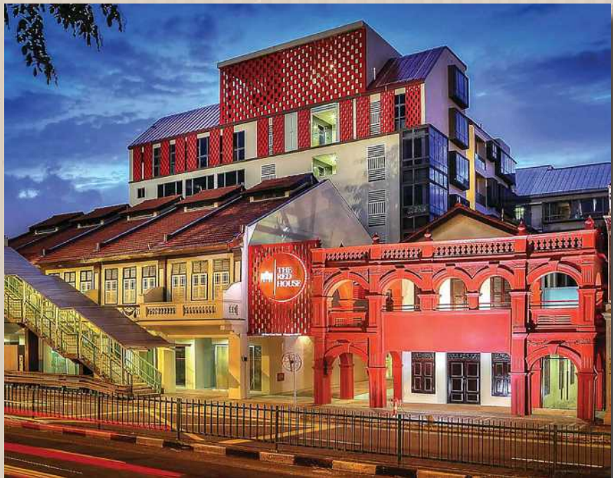
Warees Investment's signature Wakaf Revitalisation Scheme, The Red House, was bequeathed by Sheriffa Zain Alsharoff Mohamed Alsagoff. Image obtained from Warees Investments.
