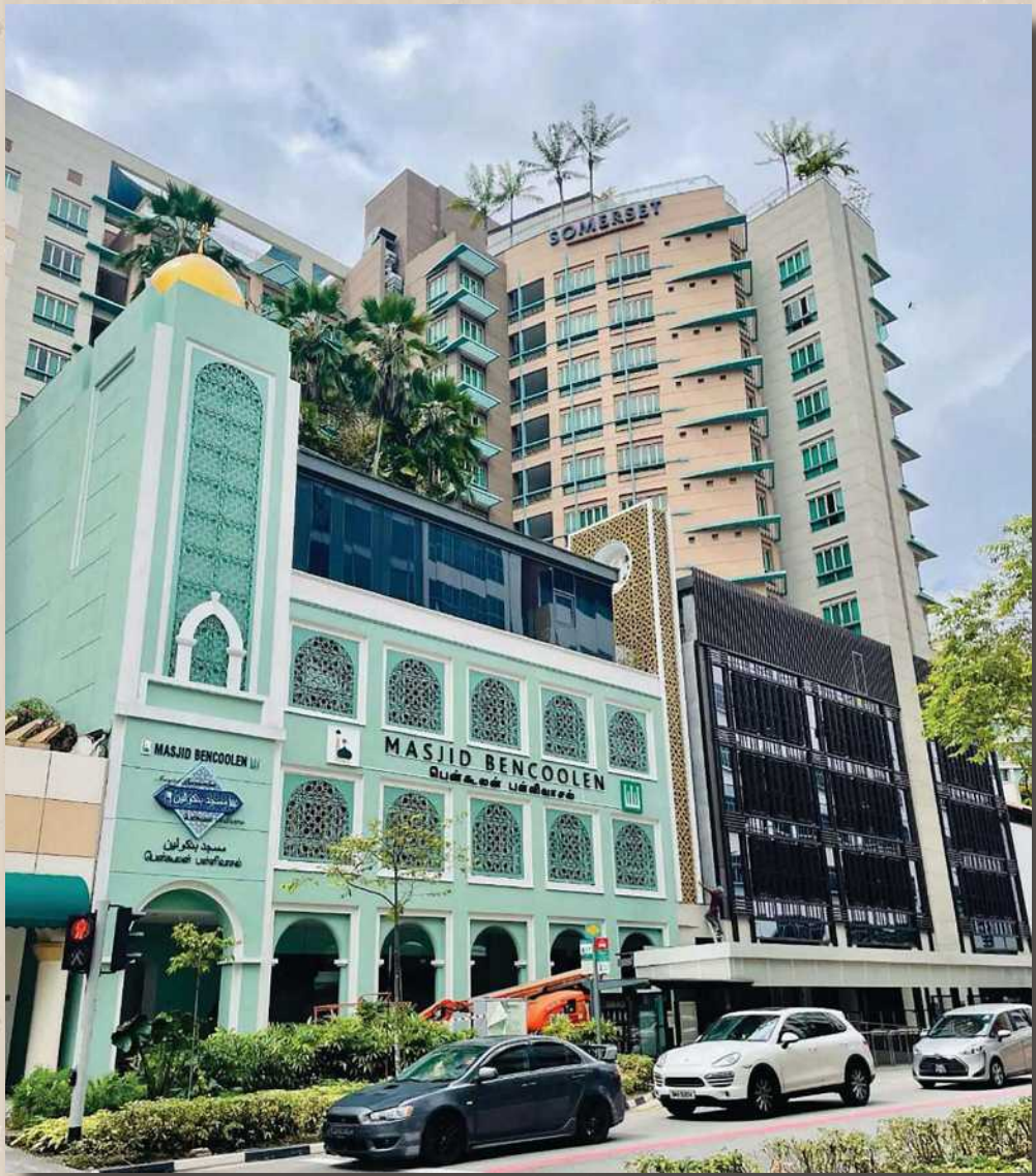
Bencoolen Mosque after redevelopment. Image obtained from Community Funds Administration, Islamic Religious Council of Singapore (Muis).
