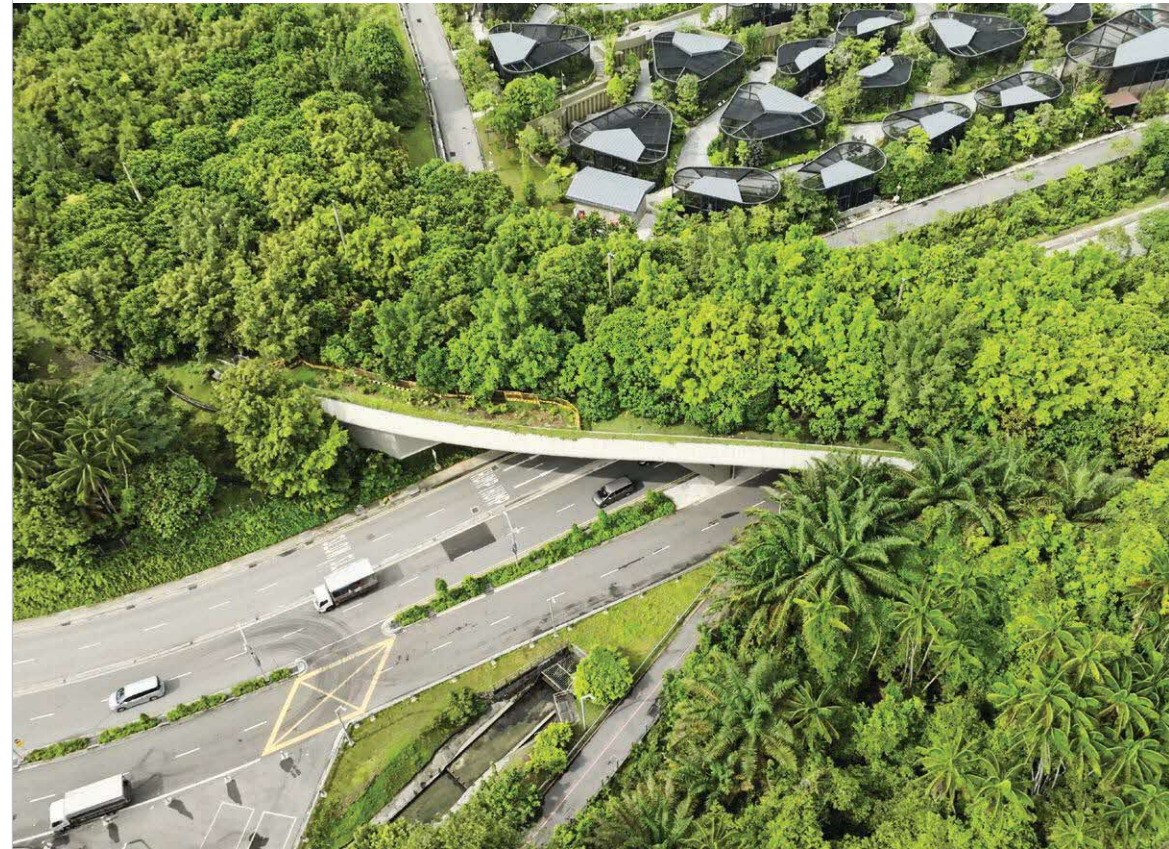
53. An aerial view of the Mandai Wildlife Bridge, taken in 2025
