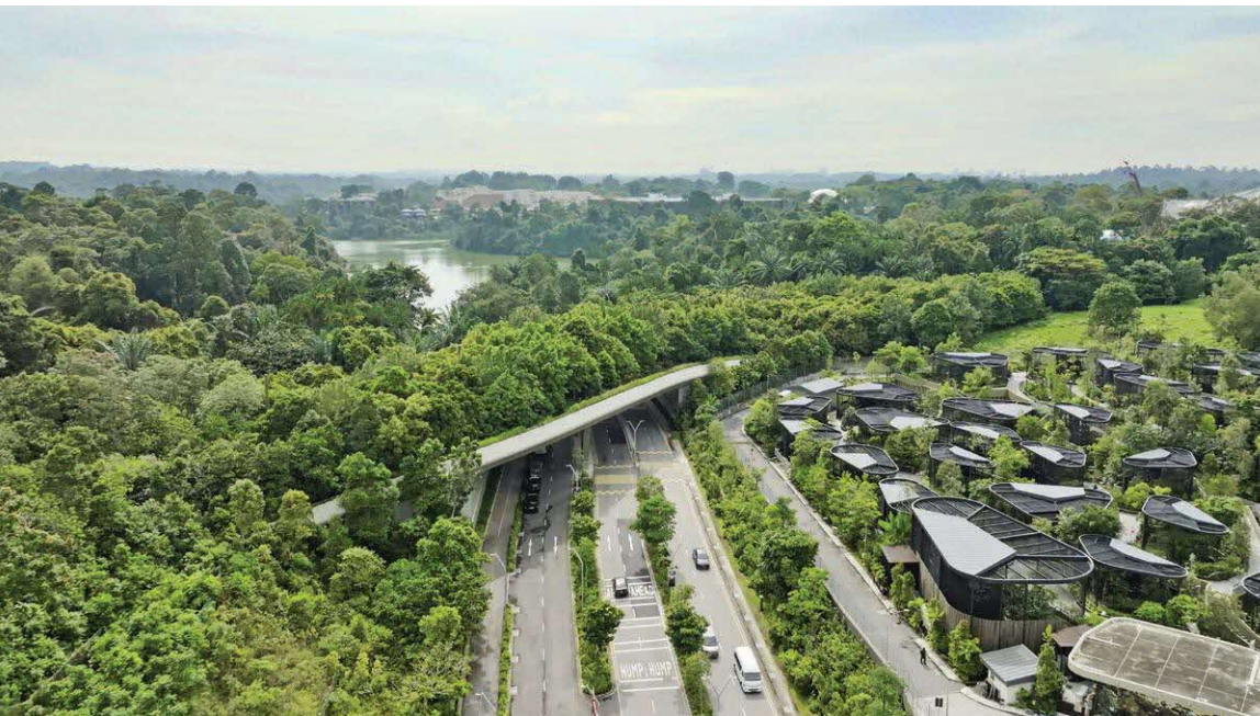
40. The Mandai Wildlife Bridge was built in December 2019 to link forest patches next to the Central Catchment Nature Reserve
