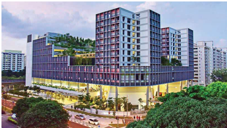
27. Kampung Admiralty, an integrated community and housing development co-located with Admiralty Place 172
