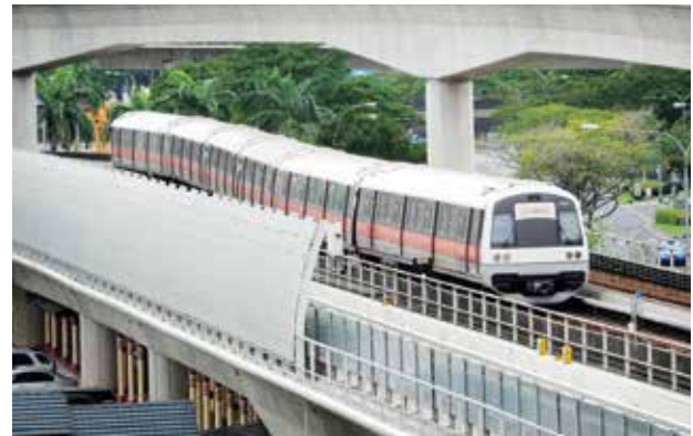
Noise barriers near Jurong East MRT Station
