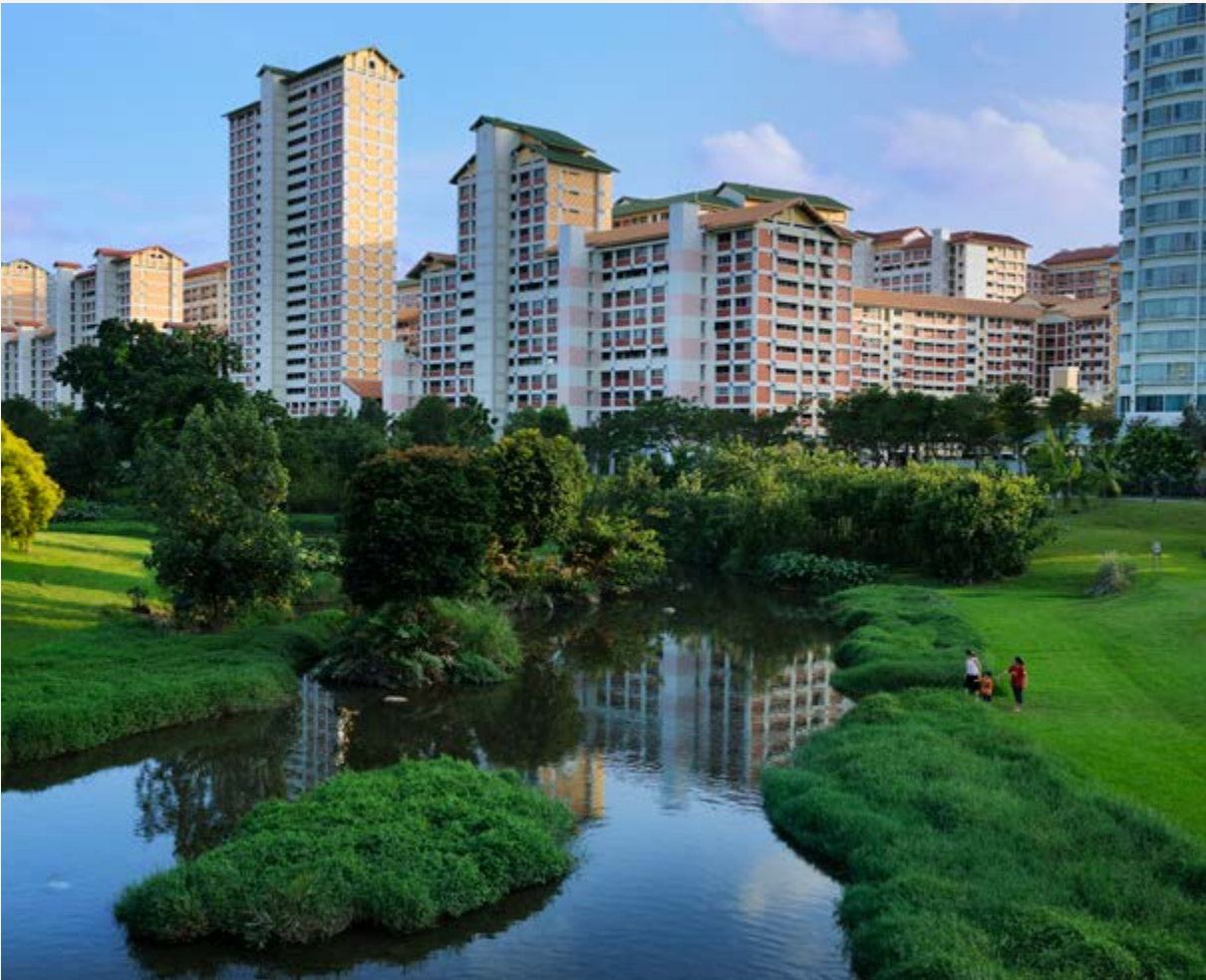
The landscape of Bishan-Ang Mo Kio Park was reconfigured to manage stormwater, prevent flooding, and support biodiversity within an urban setting.
