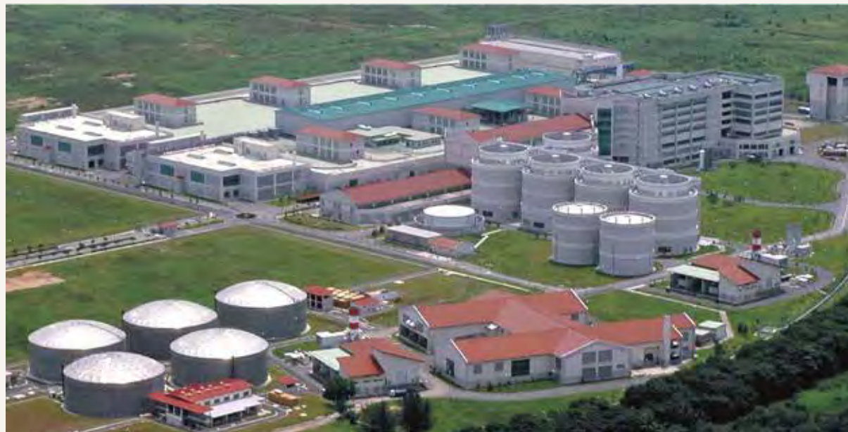
The biogas produced in the digesters at Changi Water Reclamation Plant (above) is used as fuel to either generate electricity to power the operation of the treatment facilities or dry dewatered sludge further to become dried sludge.
