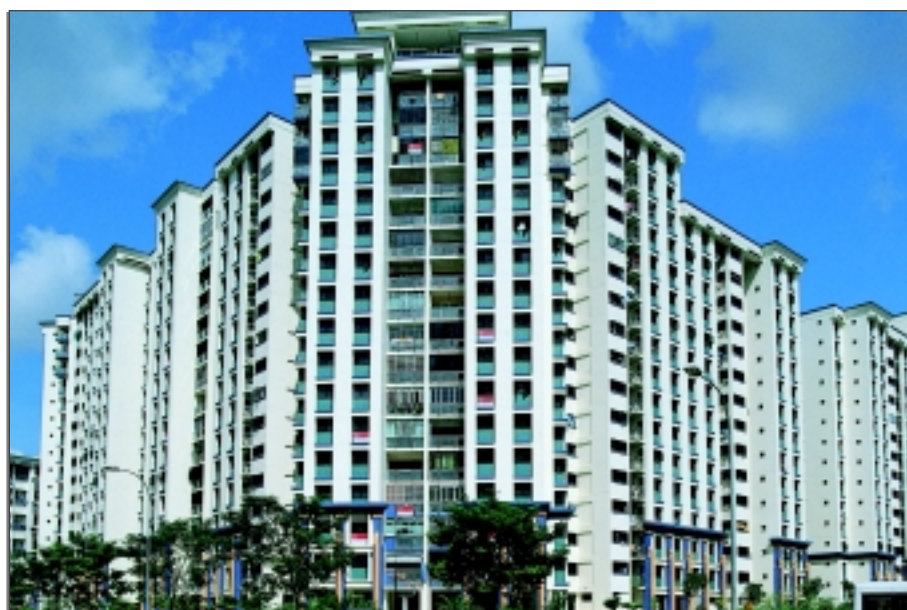
Public housing designed for optimal natural ventilation.
