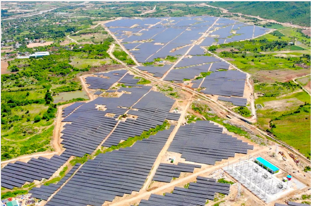
Sunseap’s 168 MWp solar farm in Ninh Thuan, Vietnam is one of the largest in the country. Sunseap and InfraCo Asia contributed three billion Vietnamese dong (S$173,749) to fund the construction of concrete roads surrounding the site. At peak construction period, the project created over 2,000 jobs, mostly for locals in the area.
