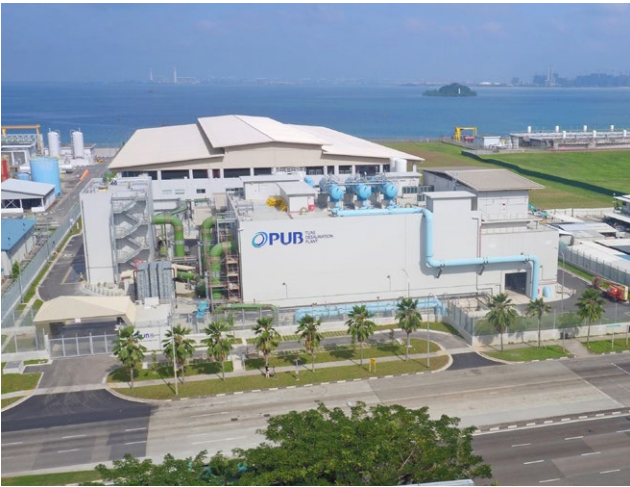
The Tuas Desalination Plant is the first in Singapore to be fitted with solar panels, with more than half of the total roof area covered by solar panels. The 1.2 MWp solar PV system will meet all of the energy needs of the plant’s administrative building.
