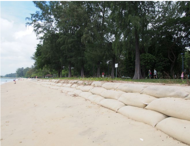
Geo-bags at East Coast Park. The geo-bags, which blend in with the beach environment, are used to prevent beach erosion while still allowing for public access.
