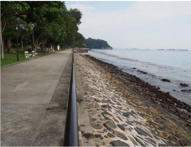
Sloping revetment at Labrador Nature Reserve. A revetment is a sloping structure built to absorb the energy of incoming waves and prevent coastal erosion.
