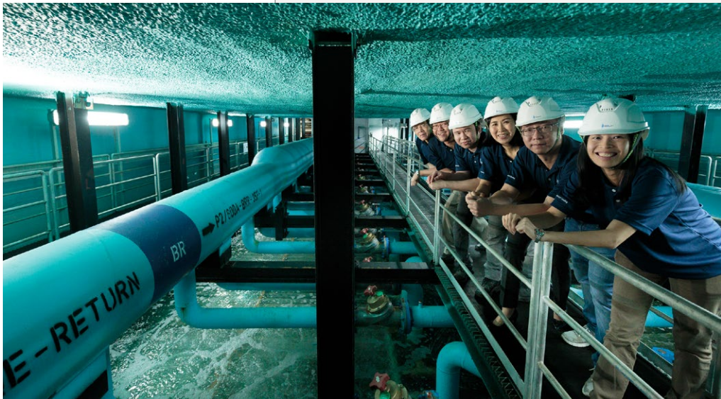
With two district cooling plants at Marina Bay Sands and One Raffles Quay, chilled water is centrally produced to support air-conditioning systems in buildings in the Marina Bay area, helping them save energy and cost.
