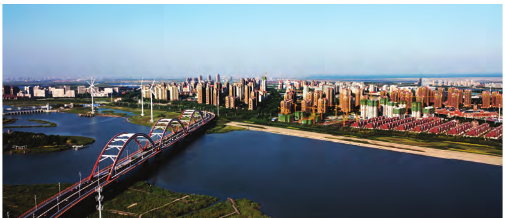
After (2015). Photo credit: Ministry of National Development
