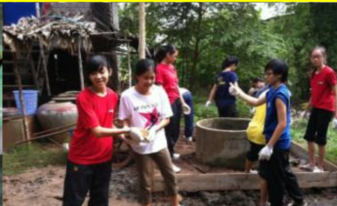
Building well pavement in Cambodia
