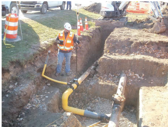
Figure 1: Surveyor recording GNSS observation on a gas main (Michigan Department of Transportation, 2015)
