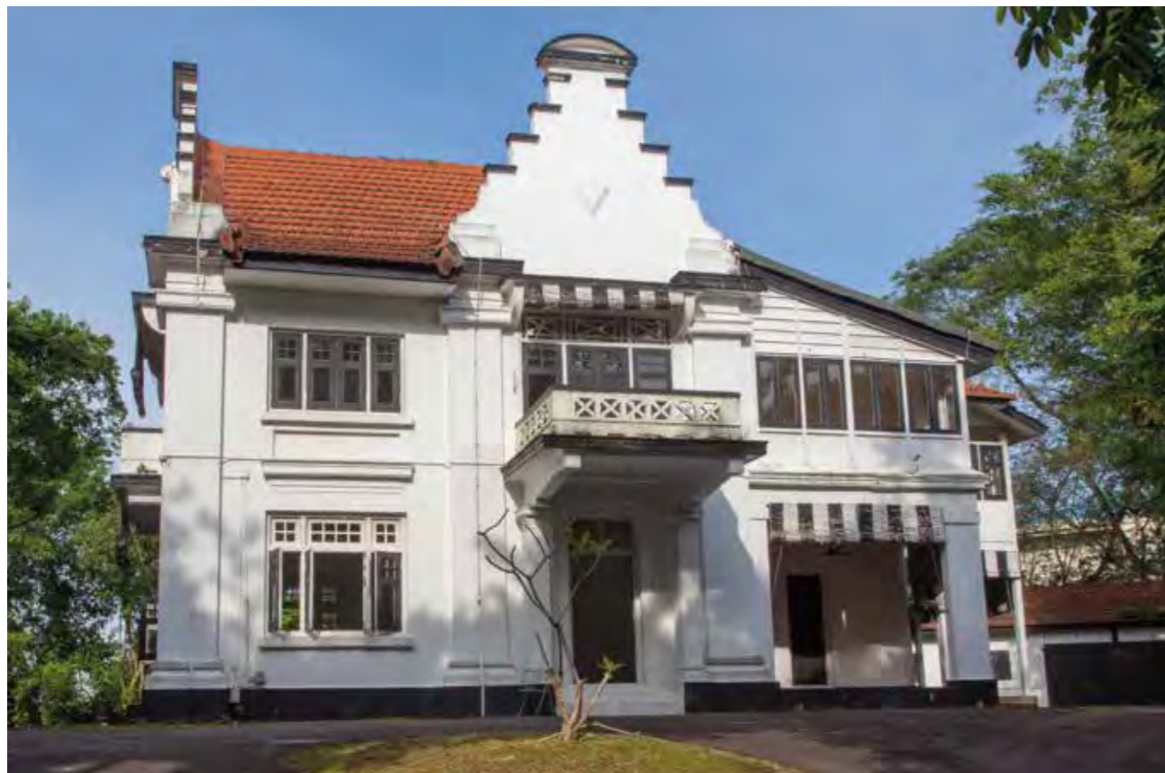
RIGHT: No. 126, one of two houses on Watten Estate Road designed by Major Percy Hubert Keys, the architect of the former Fullerton Building.
